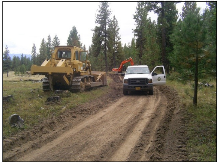
Road reconstruction project to divert road drainage away from riparian areas.
